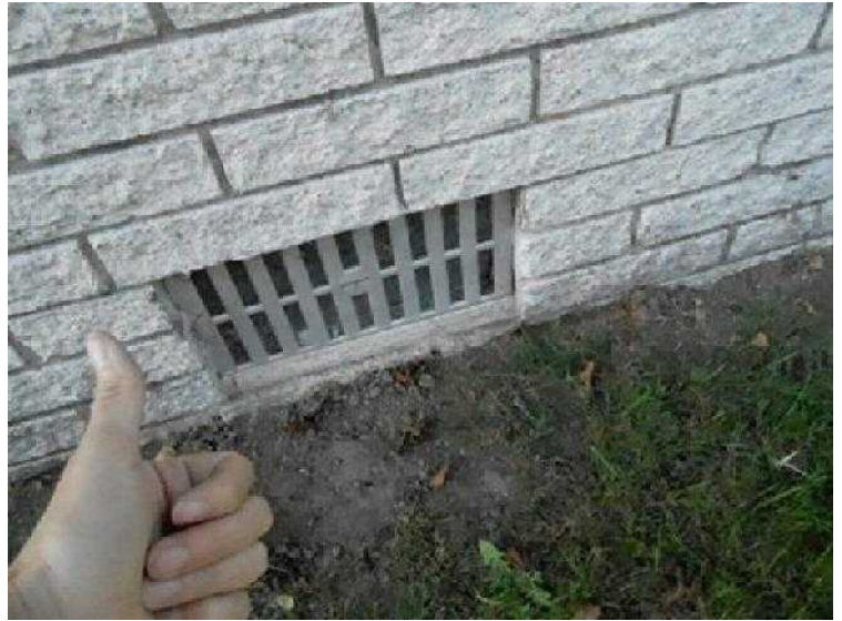
#2 This is what a typical good vent looks like. Not half buried in the ground.
