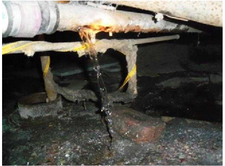
#18 Rusted out and leaking drain line pouring water into crawl space for YEARS.
