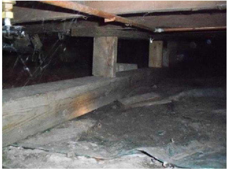
#26 They laid a 6x6 on the dirt and put cripple studs on it to support floor. Improper repair.
