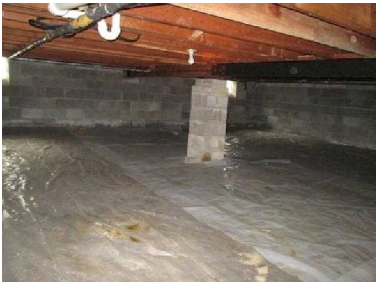
#11 Good, plastic on the ground, nice and high, vents.
