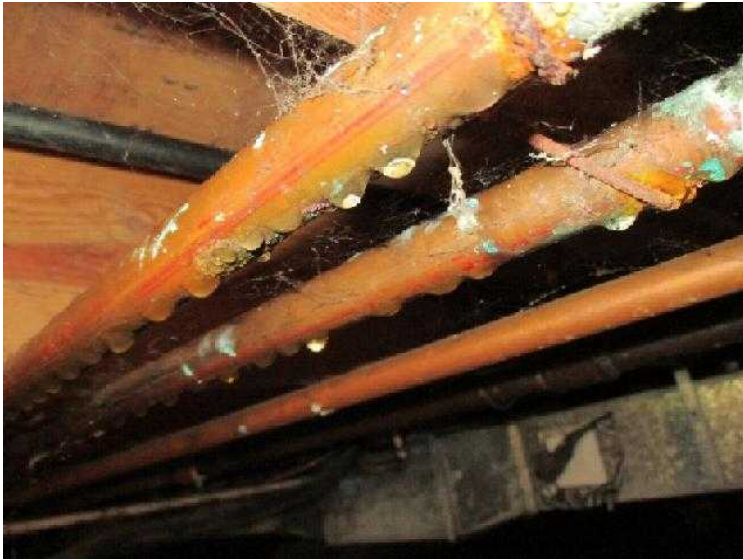
#57 Sweating water pipes can add moisture into the crawl space.
