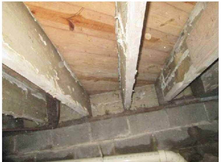
#16 Suspected mold. High humidity.
