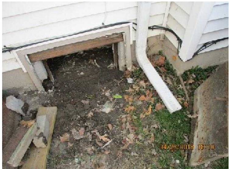
#60 Grade slants toward crawl opening. Wow. Again, why not just run the downspout right in the crawl space?
