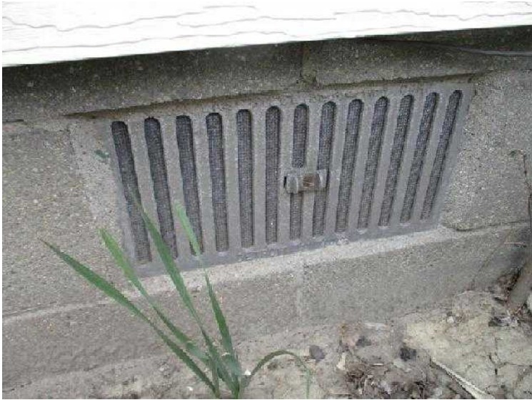
#45 Old fashioned vent. One issue they have is....the screen becomes plugged with dirt and cotton from cotton wood trees, grass clippings.
