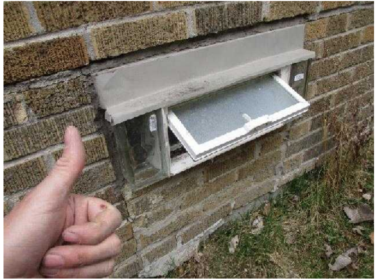
#46 Another good vent for a crawl space.
