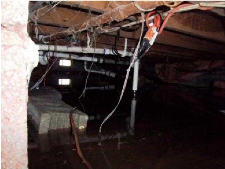
#53 This one had a sump pump but it did not work.
