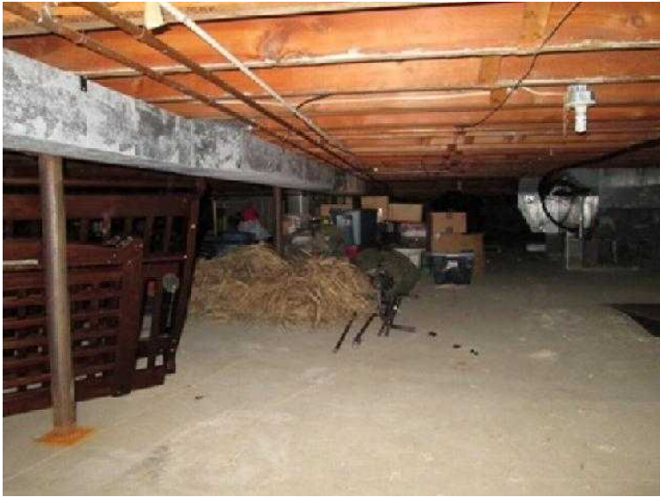
#13 Concrete floors in the crawl are great and yes, they are a vapor barrier. Again, you can cut vents in the duct work and pump conditioned air in. This will help keep it dry.
