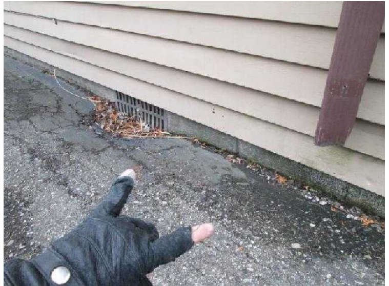
#50 The nearby downspout will ensure that lots of water will flow into the crawl space.
