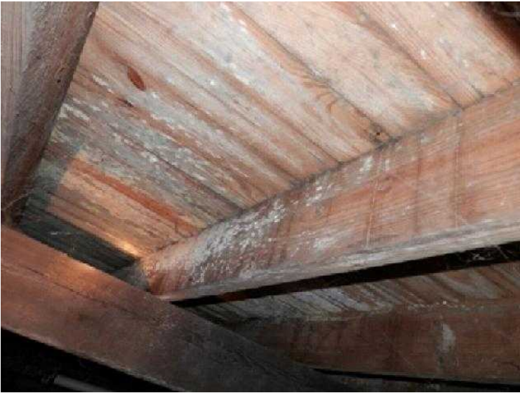
#17 Suspected mold.
