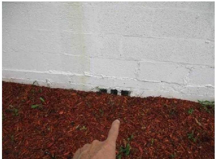
#48 Vent half buried. Lets water in.
