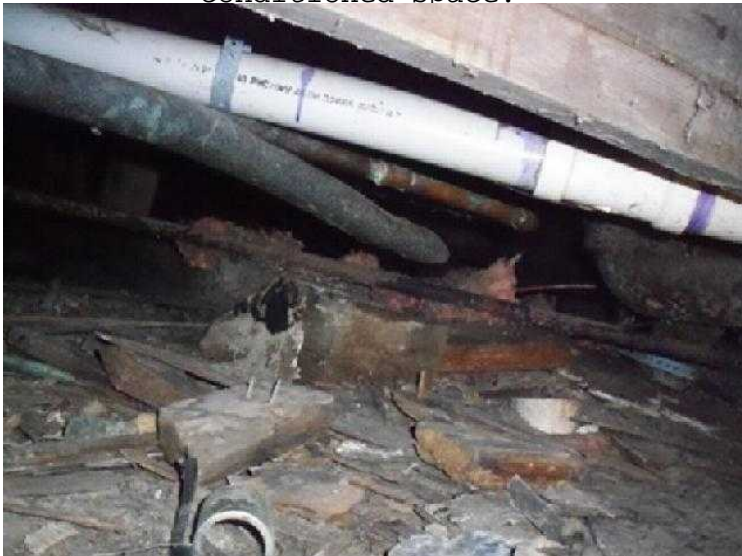
#3 Debris is dangerous, nails stick up. Wood laying on damp soil and will rot and attract wood destroying insect. Clean your crawl space out, a steel garden rake works great.
