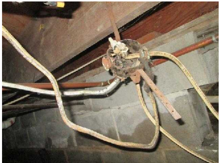
#8 Exposed live wires and wet ground.
