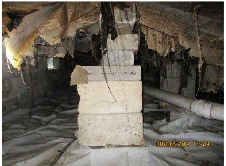
#32 Fiberglass insulation hanging down is an indication of high humidity.
