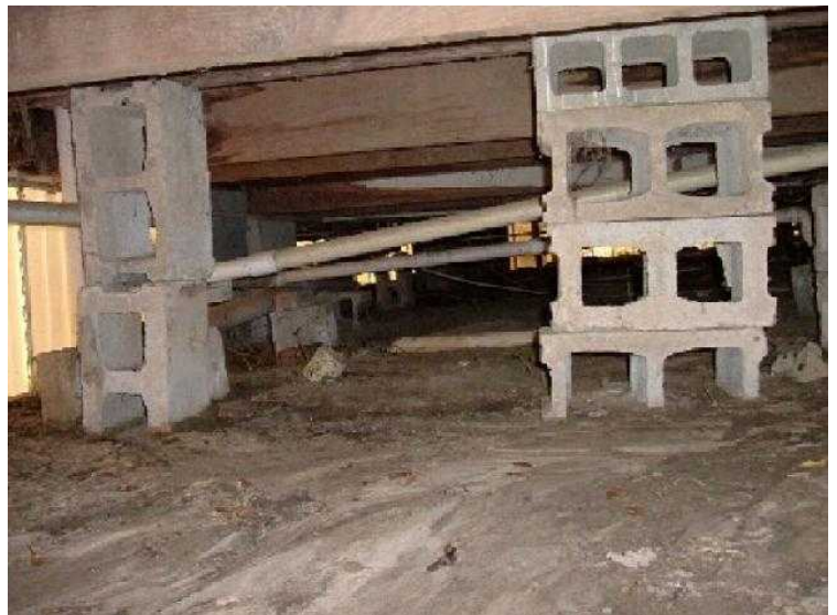
#28 Blocks installed sideways. WRONG!
