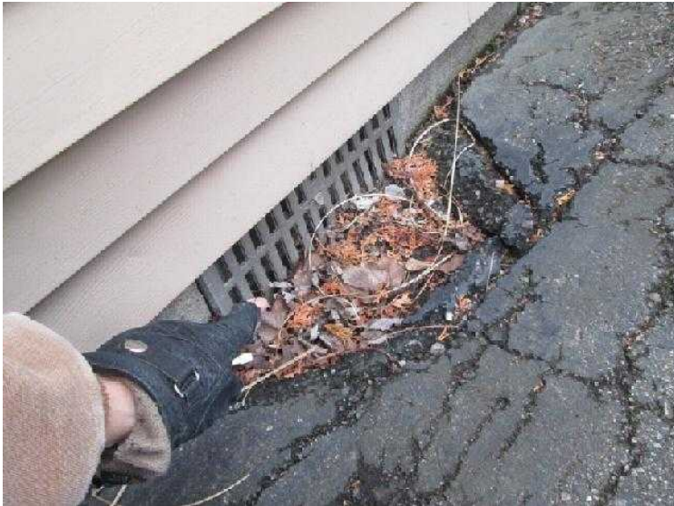
#49 This really is a funnel to let water into the crawl space.
