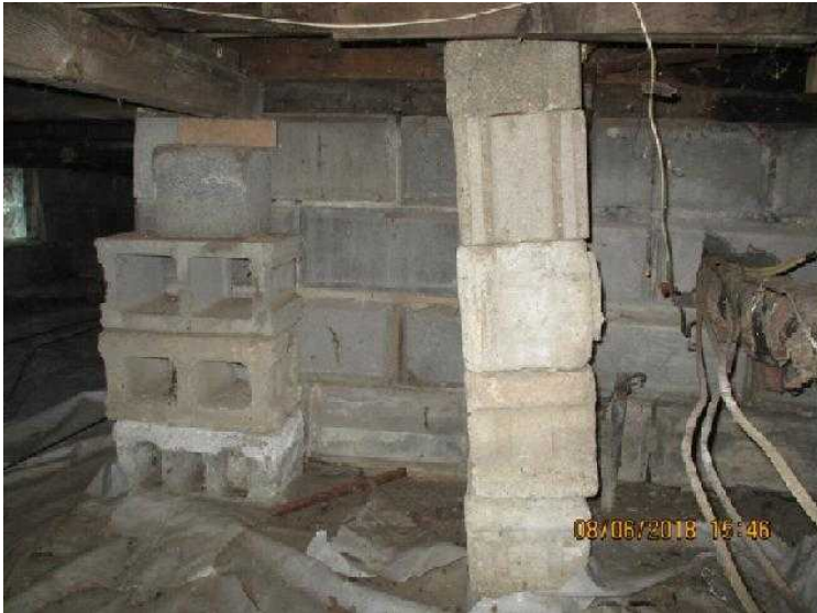
#29 Bloks installed sideways, no mortar, no footing.
