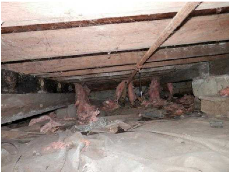
#63 Falling fiberglass insulation is an indication of moisture/high humidity.
