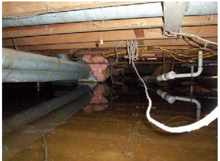
#52 Crawl space full of water. Too bad they didn't install a sump pump.
