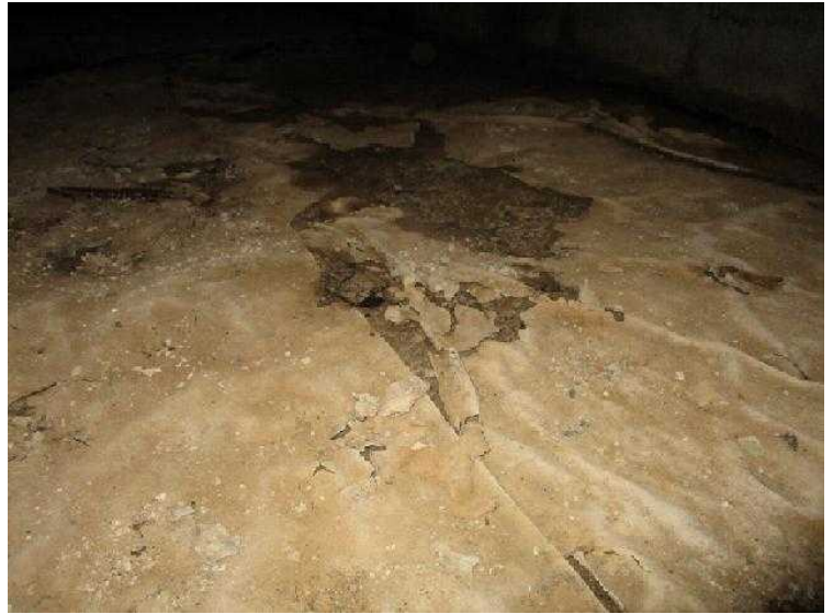
#62 Old vapor barrier. The plastic sheeting will eventually deteriorate and must be replaced. You could never see this if you put pea gravel over the entire crawl.
