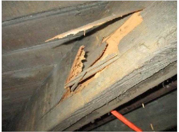
#22 Insect damage, likely powder post beetles. They leave small pin holes in the surface, but inside the wood is gone, powder, severe structural damage.
