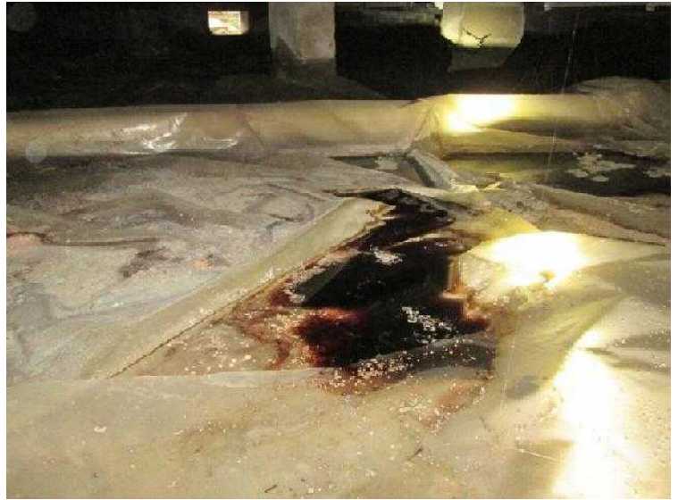
#58 Water trapped on top of vapor barrier. Water cannot soak into soil, must evaporate into air...better have vents! Fungus growing in the water.
