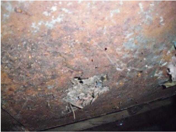
#5 Rusted out duct work. A sure sign of dampness in the crawl space. Great path for mice to get into house.
