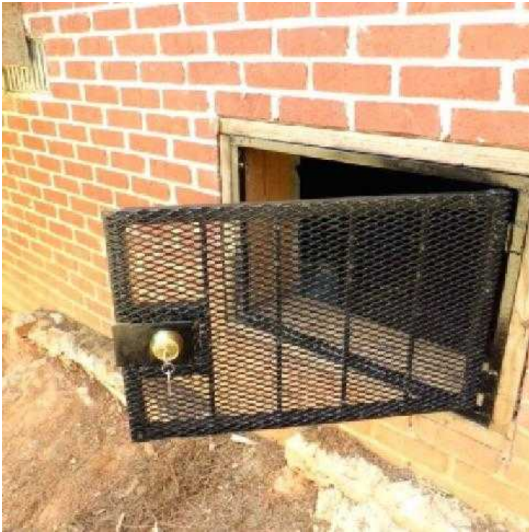
#41 Access door is also a VENT. Nice custom job. The owner filled the gap with ridged foam insulation in the winter.
