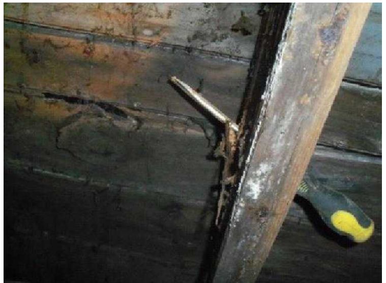
#20 Wood was so rotten I could push a screwdriver all the way through it. This was an older home, on a canal in Harrison Twp. MI.
