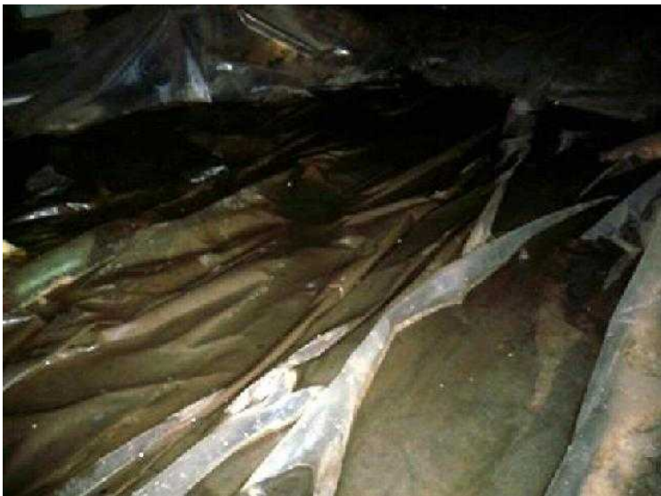
#55 If water ever gets on top of the vapor barrier, from a leaking pipe, overflowing toilet, leaking tub trap, the vapor barrier becomes a swimming pooling liner and holds water in crawl.
