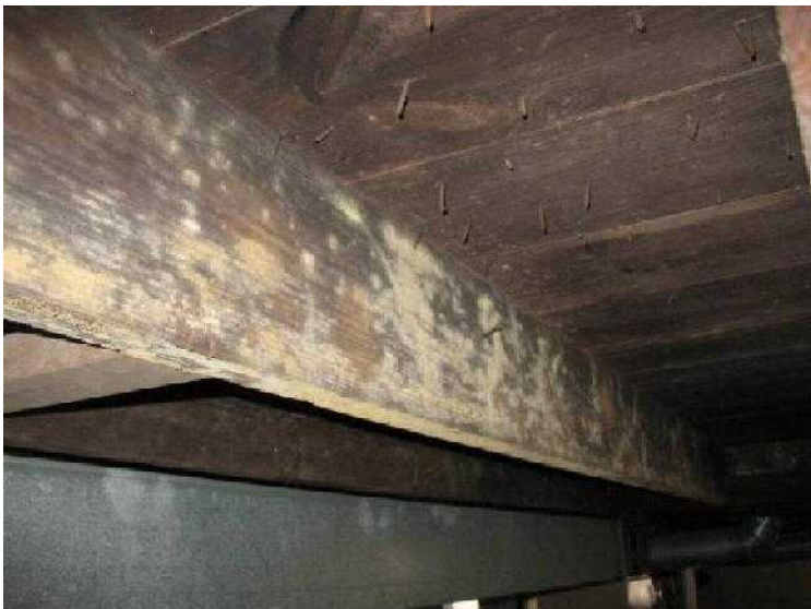
#15 Suspected mold. High humidity in crawl. Cutting a couple of vents in the duct work may have prevented this.
