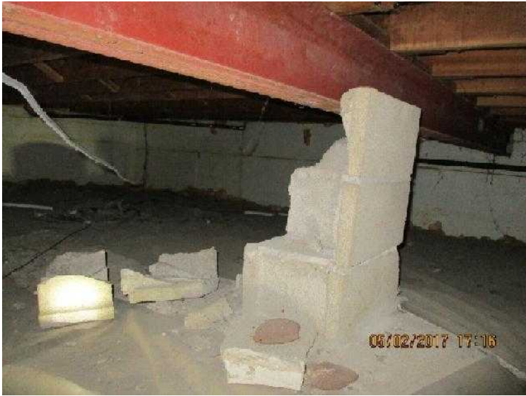
#25 Block column split off. This is unusual.
