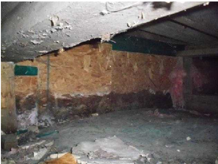
#27 OSB plywood touching soil and soaking up water. This is on one of those "pier foundations" where the house sits on blocks, like a trailer and there is a skirt around the house.
