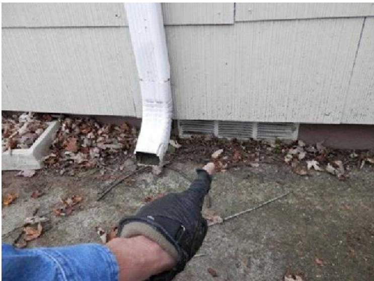
#51 Negative pitch on dirve, vent at grade. Why not just turn the elbow around and dump the water directly into the crawl space?
