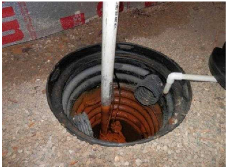
#36 Nice sump pump in crawl space. Notice the orange substance. That is "iron fungus"....or maybe just clay, or both. Causes sump pump to fail sooner.
