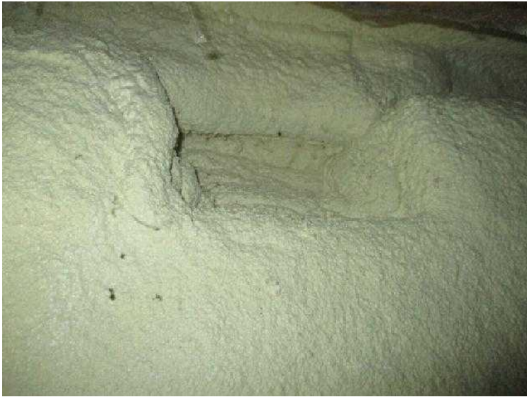
#9 Spray foam over the vent in the foundation. Don't let anyone eliminate your foundation vents. You may need them.
