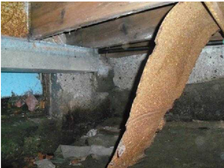
#7 Cold air return rusted out at nails and fell.
