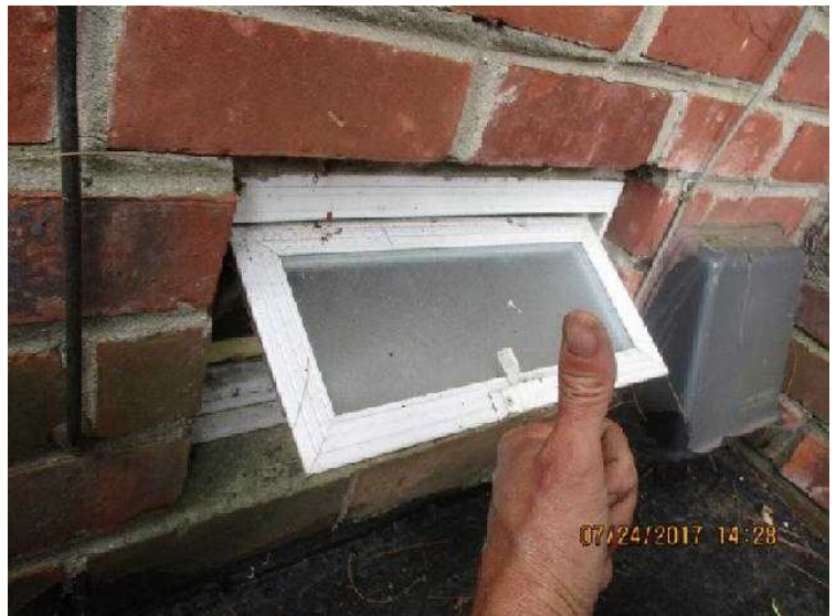
#44 This is a GREAT idea. Glass block window vent in a crawl space. Install backwards and upside down. Opens from the exterior, lets light in.
