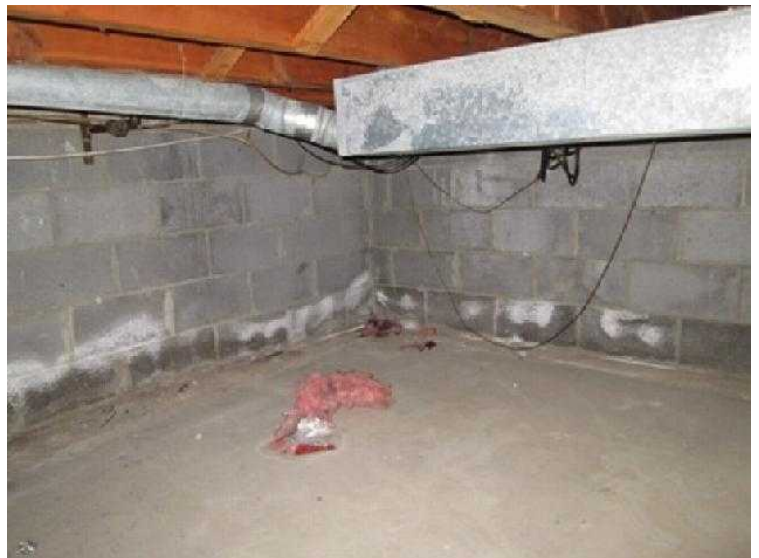
#12 Nice high crawl space. But water marks on walls indicate some moisture. Vents can be cut into the duct work to pump conditioned air into the crawl.
