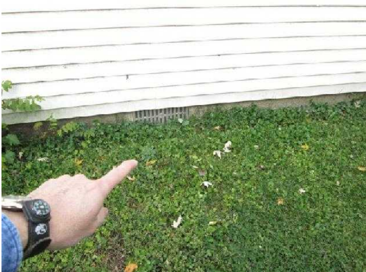
#43 Vents at grade level become a funnel and let water IN the crawl instead of letting humidity out.
