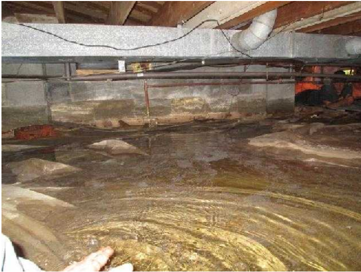
#61 Naturally it was full of water. Pond on top of vapor barrier. Now the vapor retains water in the crawl rather than keeping it out.
