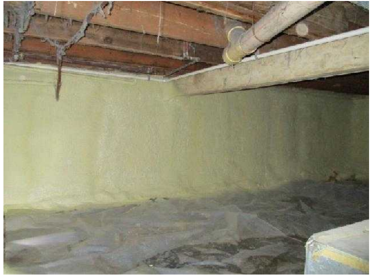
#10 This is what a good crawl space looks like.
